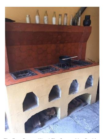
The Four-Burner, Wood-Fire Stove with a Beehive Oven
